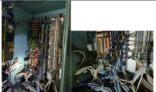
No.2 Several disconnected cables and bridges were found in the engine room inside the control box (ballast water management system). The system has been manipulated. (Ground for Detention)
