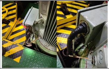
No.4 Found an manipulation (flying additional relay) in the RWO WATER TECHNOLOGY switch box.
