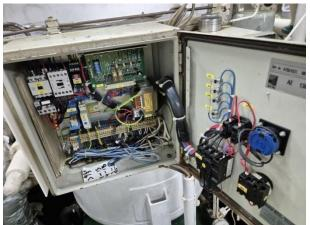
No.5 Found in steering gear (contactor cabinet warning box) a flying relay. **(Ground for Detention)**
