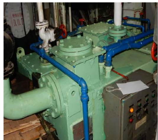
Top of sewage treatment plant leakage
