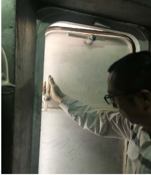
E.R escape door locked from outside
