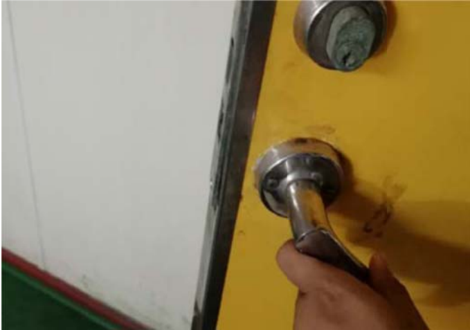
Crew smoking room door not closed tightly( Oil Tanker)
