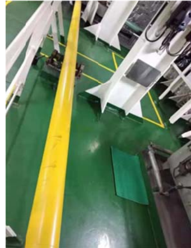
Steering Gear room floor too oily
