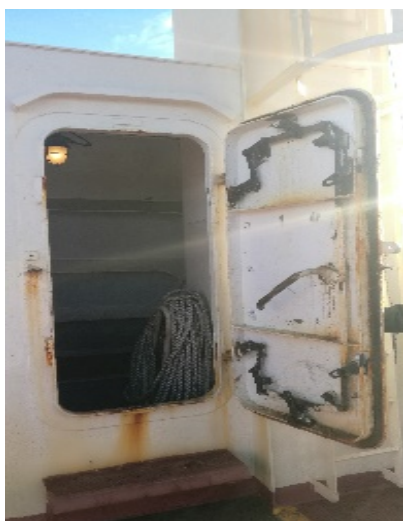
The store room door at forecastle can not be closed properly
