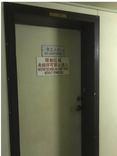
Automatic closing fire door (after rectification)
