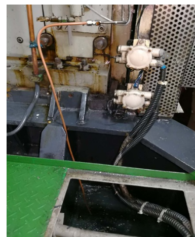
Copper tube replaced
