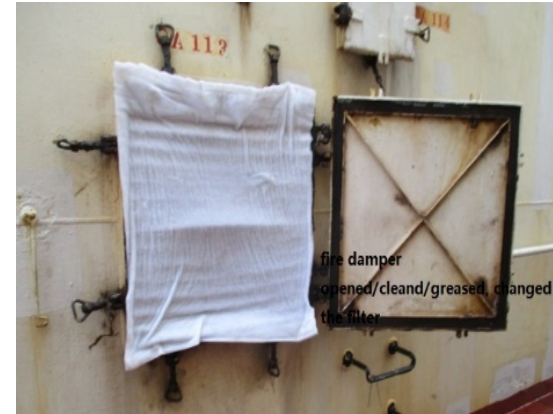
Shutter for ventilation opening in engine room cannot be closed
