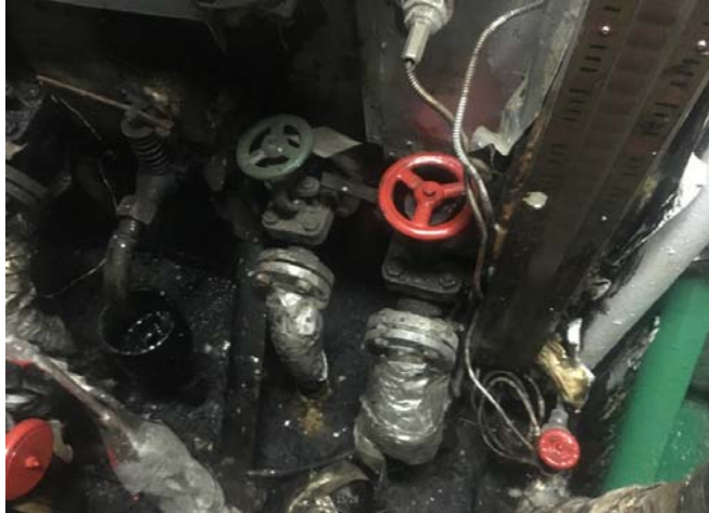
Quick closing valve of fuel oil tank did not work
