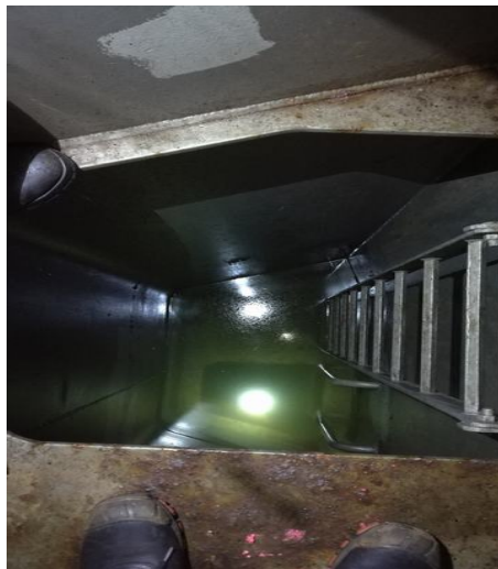
Pipe tunnel and cargo holds ingress due to ballast pipe broken.
