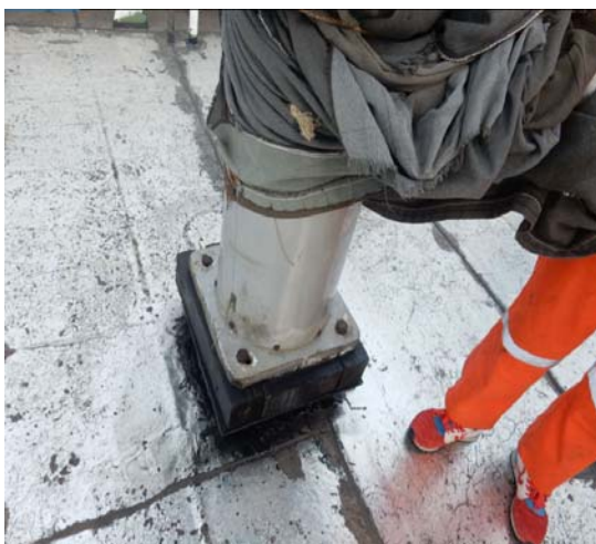
Wooden base of magnetic compass on flying bridge deck rotted.
