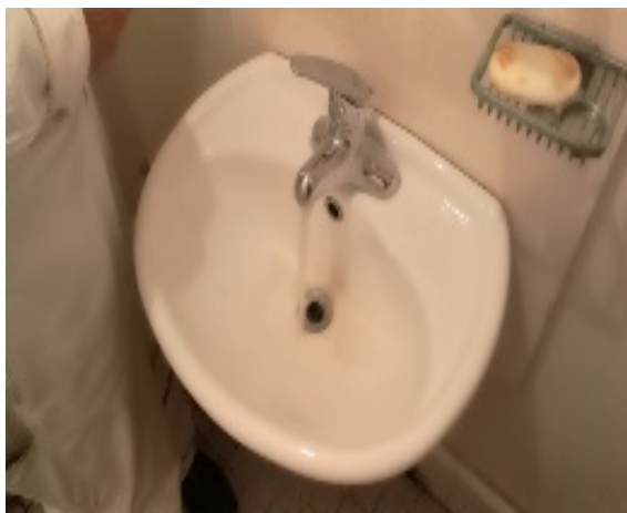
Several taps (wash bin) disconnected.
