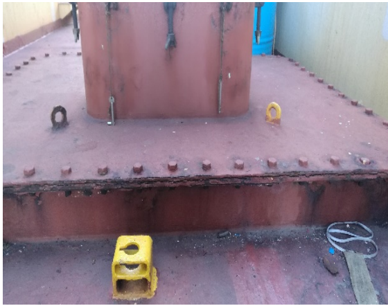
The large store cover ER showed not be weathertight/ watertight.
