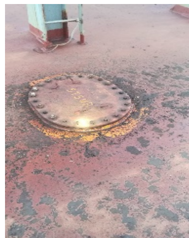
Ballast tank manholes were closed watertightly
