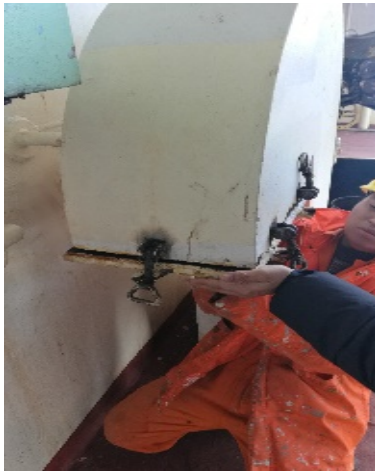
The cover plate of the gooseneck ventilator cannot be closed
