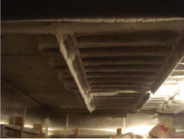
Evaporator in meat and fish room is frozen.
