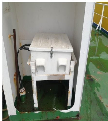
Battery room charger not properly fixed
