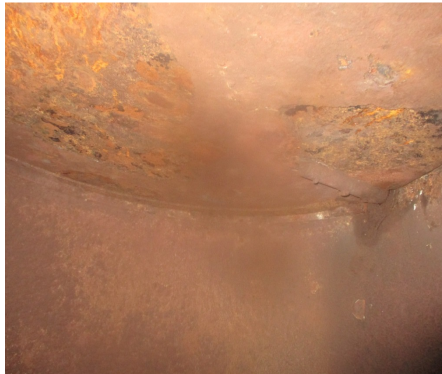
Engine room fire dampers unable to be effectively closed locally and from remote
