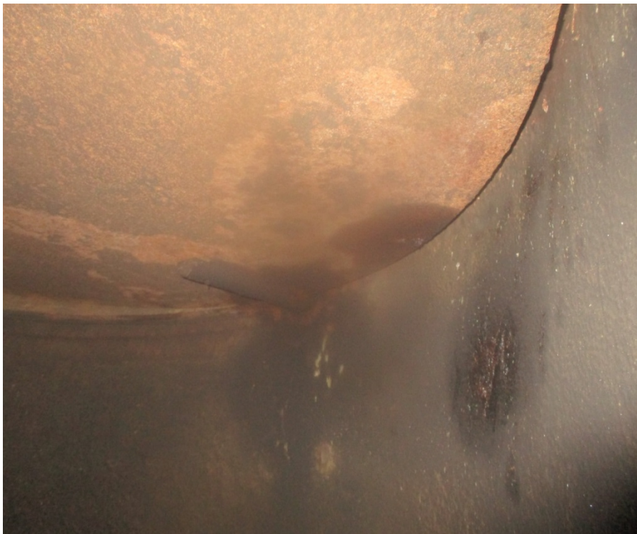
Engine room fire dampers unable to be effectively closed locally and from remote
