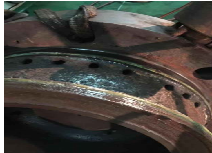
M.E. cylinder water leakages
