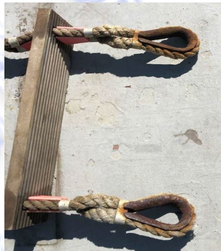
Figure 2 Example of corroded end point thimbles (protective rings)
