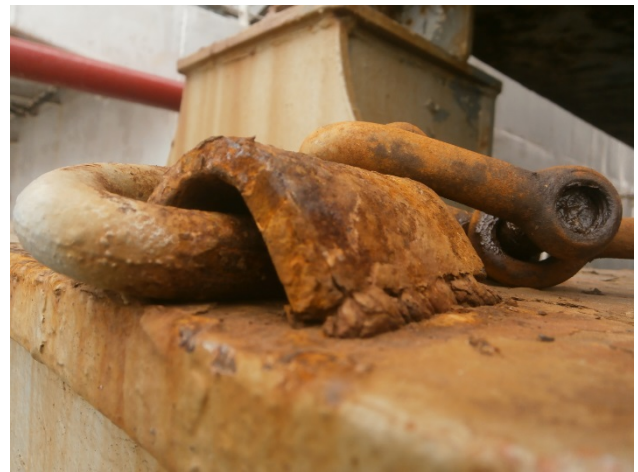
Serious Corrosion and Damage of Securing
