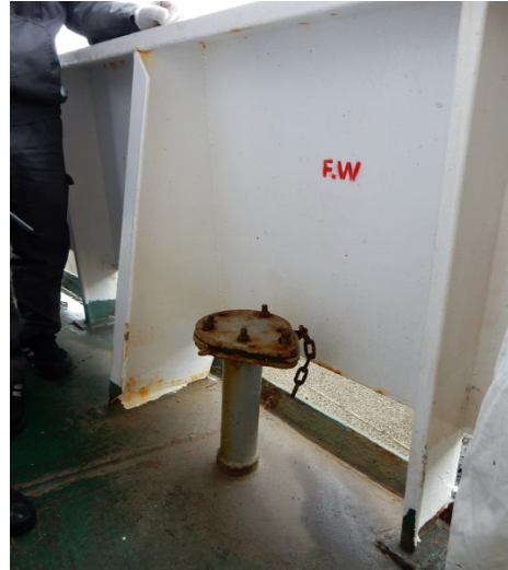
Serious Rusting of Water Filling Nozzle Cover of Fresh Water Tank
