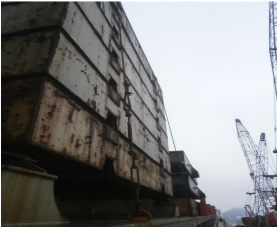
Portable Covers Securing Not Meeting Requirements
