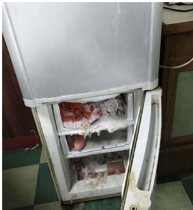
The refrigerators in senior officers' rooms and pantry are freezing
