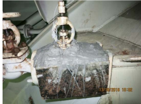
The sewage discharge outboard valve is holed (temporary plugging with iron cement has been done)
