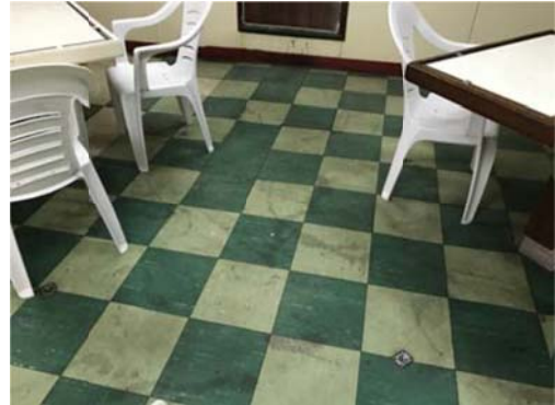
The number of chairs in dining room is insufficient. Some floor have cracks and the floor is dirty
