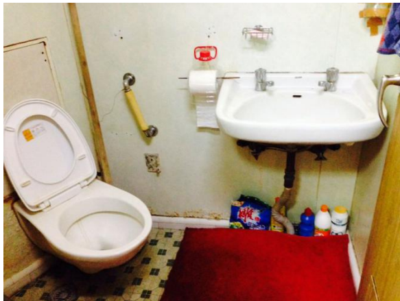
The sanitary fixture is damaged and in a mess
