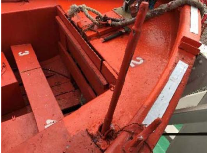
The cover support of lifeboat is seriously corroded, and the fixed pin and connecting rod with defects
