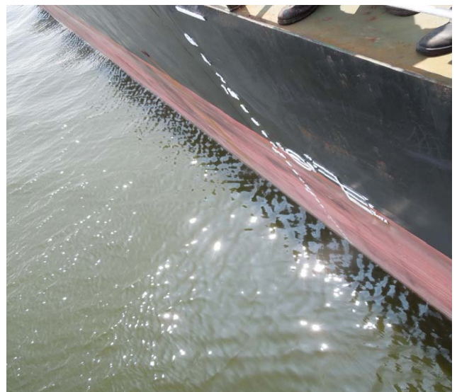
Load line mark isn't clear (repainted)
