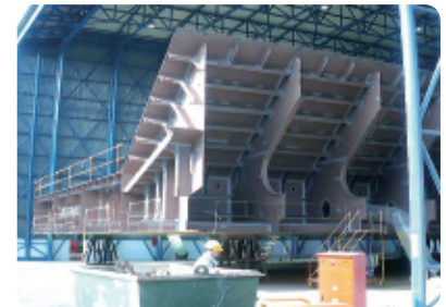
block in Coating Workshop to be Coated
